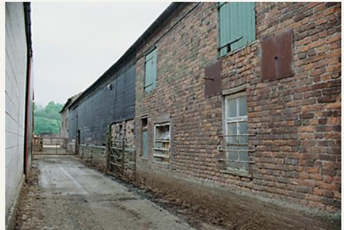
on a stone plinth and has a slate roof. It has a rectangular plan with six bays, and contains a large wagon entrance. This is a structure of high quality and has been little altered.
