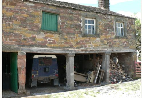
It has a long rectangular plan, with chimney stack and external steps to a loft at the right end. The front wall is of coursed roughly squared red sandstone with larger quoins. The right half of the ground floor is a continuous opening, there is a re-used lintel a bridging beam supported by 2 tapered hexagonal stone columns.
