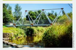
The bridge is based on a structure invented by the Scottish Engineer Charles Inglis at the turn of the 20th century. The portable bridge was specifically developed for the British Army during WW1. It was designed to enable troops, artillery and tanks to continue to advance, and to be sustained with supplies. This type of bridge played a strategically important role in 1918, enabling the Allies' sustained momentum for the advance which ended the war. Speed was vital
